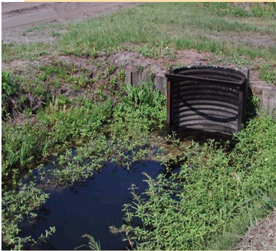
Figure 9. With subsurface (seepage) irrigation, water levels in the field are controlled by removable boards. Photograph by: Eric Simonne.
