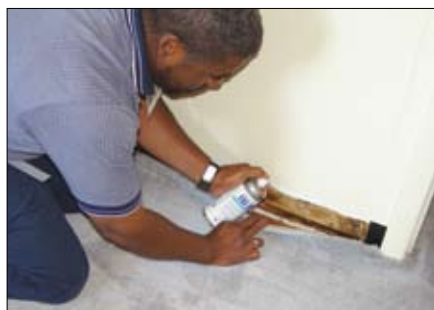
Fig. 3. Treating sill plate to tack strip with Tri-Die (Whitmire Micro-Gen) after removing baseboards and lifting carpeting in a bed bug-infested apartment. (Photo: W. Walker)
