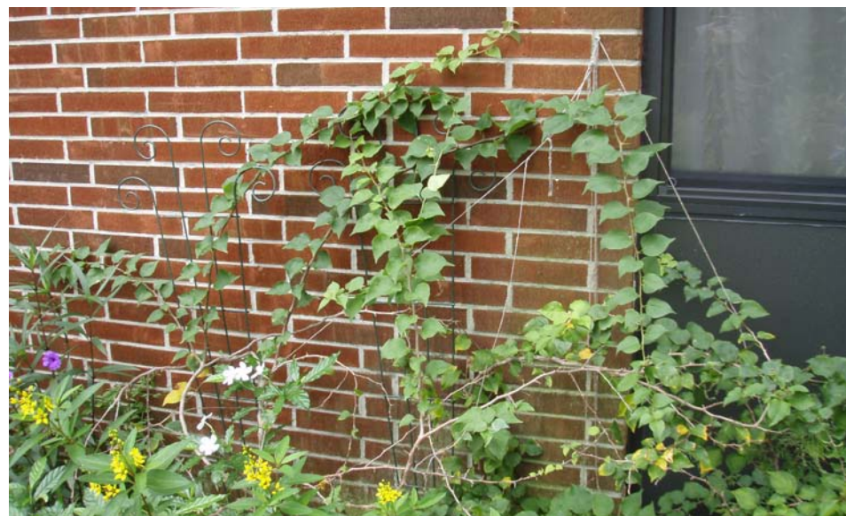
Figure 7. Vining plants can give insects access into buildings.
