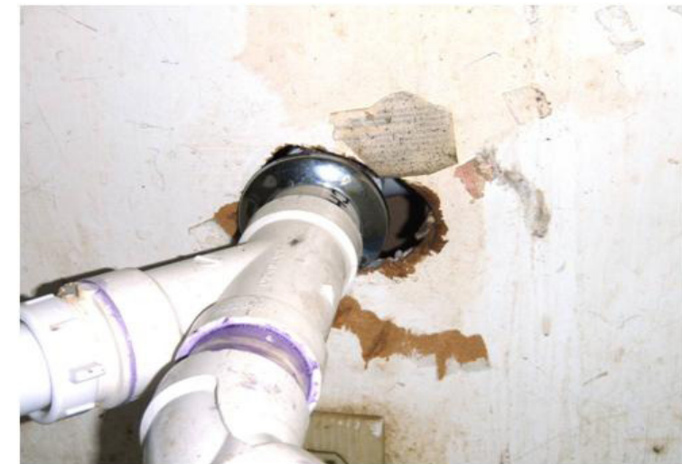
Figure 2. An improperly installed escutcheon plate can be repaired by the DOHRE Maintenance Section.
