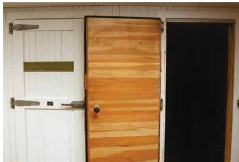
Cool storage facilities are essential for a berry operation since berries must be cooled immediately after harvest to prolong shelf life. Photo by Luke Freeman.
